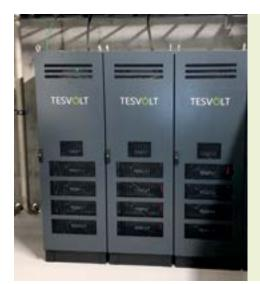
"TESVOLT battery storage systems are the only storage systems on the market that can be fully charged and discharged twice in one day and still maintain their long service life. Many suppliers only enable one storage system charge and discharge cycle per day, which wouldn't have worked for the salmon farm." Jonas A Kverneland, Technical Manager of Kverneland Energi
